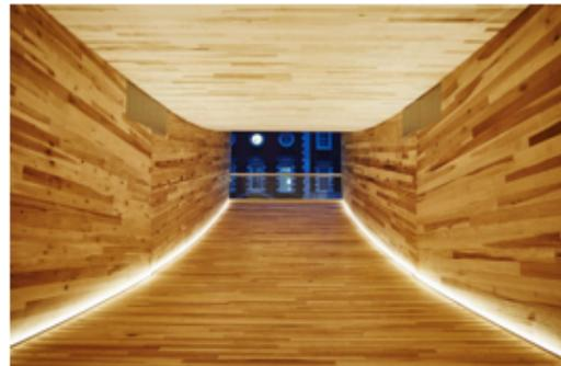
The Smile is one of the Festival's Landmark Projects, which can be inhabited and explored by the public. The spectacular, curved, tubular timber structure measures 3.5m high, 4.5m wide and 34m long and is effectively a beam curving up at both ends. Showcasing the structural and spatial potential of cross-laminated American tulipwood, Alison Brooks' concept is the first ever 'mega-tube' made with construction-sized panels of hardwood CLT.
